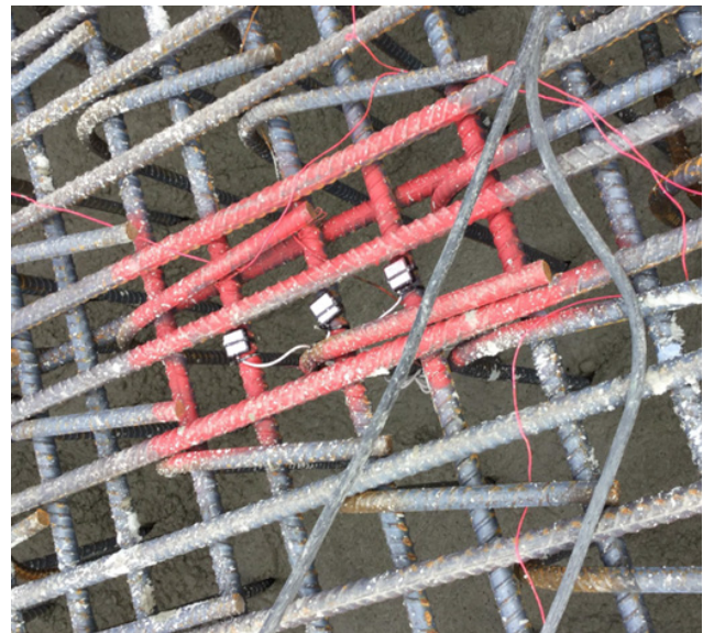
Fig. 2.7.54: Temperature sensors can be used to monitor concrete curing and estimate the in-place concrete strength. (Image courtesy of Conco.)
