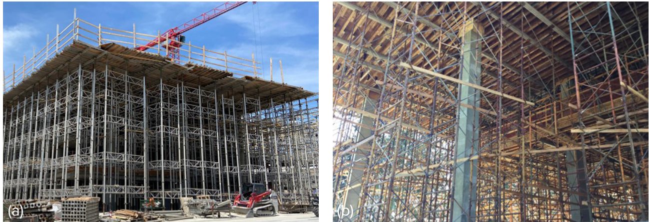
Fig. 2.6.26: Examples of high shoring. ((a) Image courtesy of Ceco Concrete Construction. (b) Image courtesy of Conco.)
