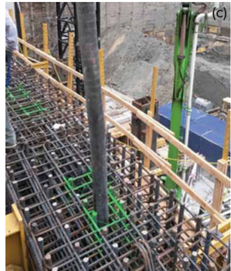
Fig. 2.7.34: Images from “ Reinforcement Congestion in CIP Concrete ” illustrate the need for pump hose and vibrator access zones: (a) schematics demonstrate the reasons for access; (b) access zones in a mat are marked in pink paint; and (c) access zones marked in green paint (spaced 10 ft apart over the top of a congested shear wall).
