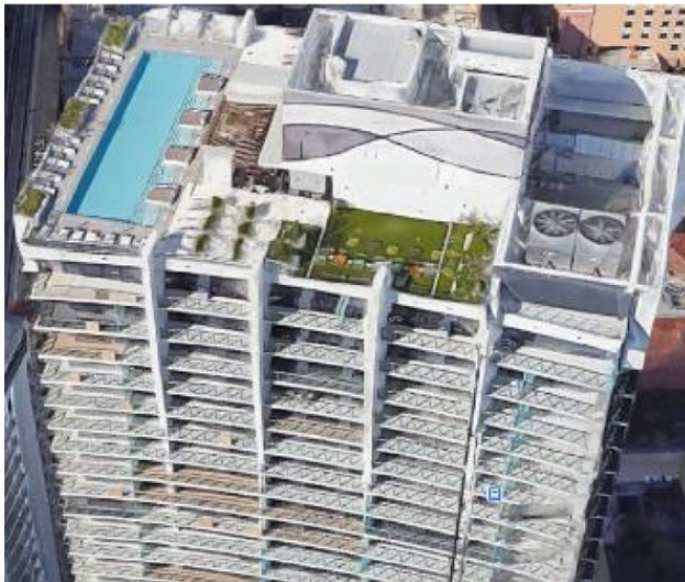
Fig. 2.6.44: A roof structure with a swimming pool, green roof, and mechanical equipment. High dead loads such as these may require a heavy structure that must be supported by multiple levels of reshores. (Image courtesy of Ceco Concrete Construction.)
