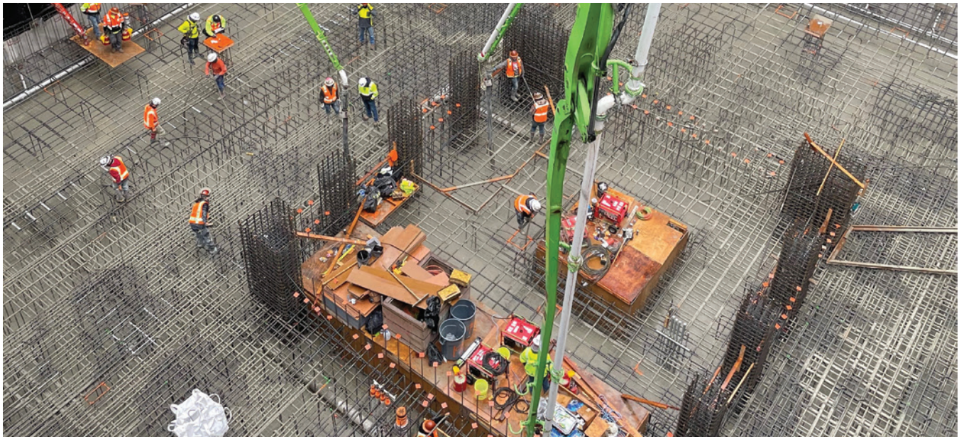
Mat pour. (Image courtesy of The Conco Companies.)
