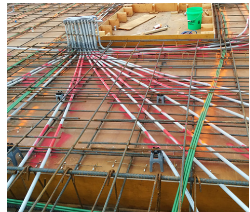
Fig 2.7.39 Electrical conduit should not impede PT strand profiles, (Image courtesy of Amsysco.)
