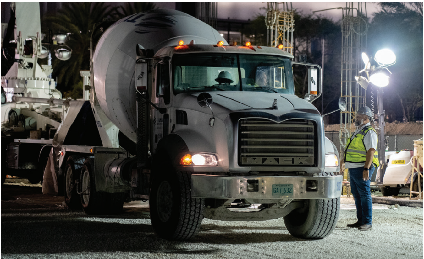
Miami World Tower. (Image courtesy of Ceco Concrete Construction.)
