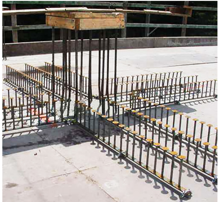
Fig. 2.7.13: Double-headed stud shear reinforcement (stud rails) can allow slabs to be constructed without drop panels. (Image courtesy of CRSI.)
