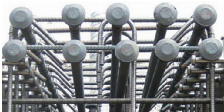
Fig. 2.7.32: Headed reinforcement can help avoid congestion and ensure adequate embedment to develop bars. (Detail source: STRUCTURE Magazine, May 2011, “Tips for Designing Constructible Concrete Structures, Part 2.” Image courtesy of Headed Reinforcement Corp.)
