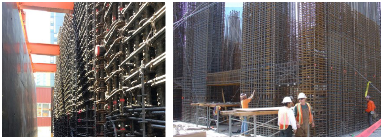
Fig. 2.6.46: High-density wall reinforcing creates challenges for workers. Wall reinforcing must allow sufficient space between bars to accommodate form ties. (First image courtesy of Conco; second image courtesy of Ceco Concrete Construction.)
